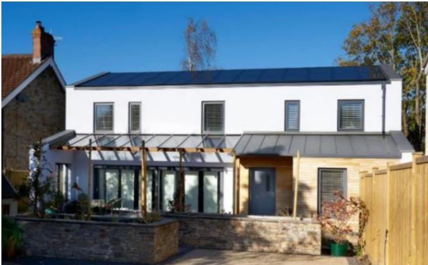
Passivhaus Plus detached home in Bristol. Reported an EUI of 30 kWh/m<sup>2</sup>/yr\* and solar generation of 40 kWh/m<sup>2</sup>/yr\* from 2019-2020.
