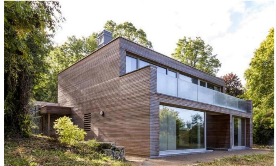
Passivhaus Plus detached house in Buckinghamshire. Reported an EUI of 25 kWh/m<sup>2</sup>/yr\* and solar generation of 18 kWh/m<sup>2</sup>/yr\* from 2019-2020.
