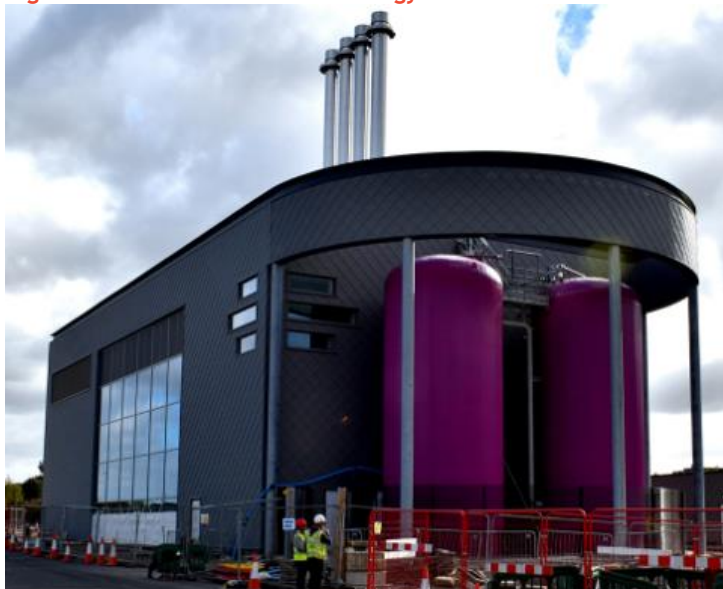
Figure 28: Gateshead District Energy Centre
