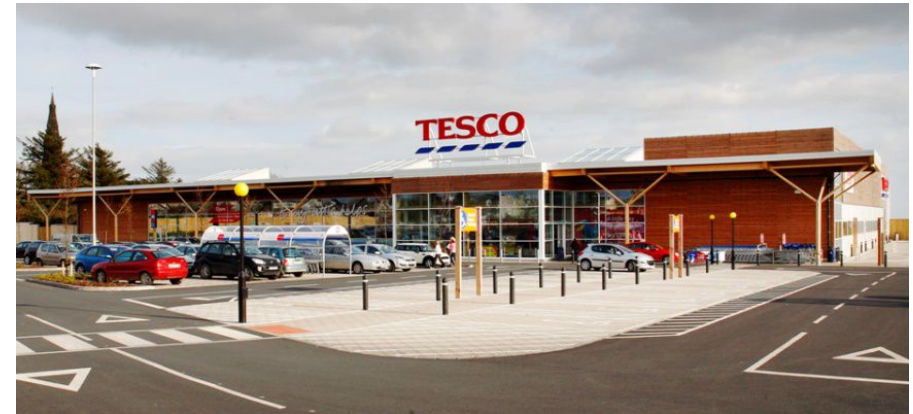
The first Passivhaus supermarket in the world was created in 2008 in Tramore, Ireland. It has solar photovoltaic panels and a ground source heat pump that provides water heating from waste heat taken from the cooling cabinets. © Joseph Doyle Architects
